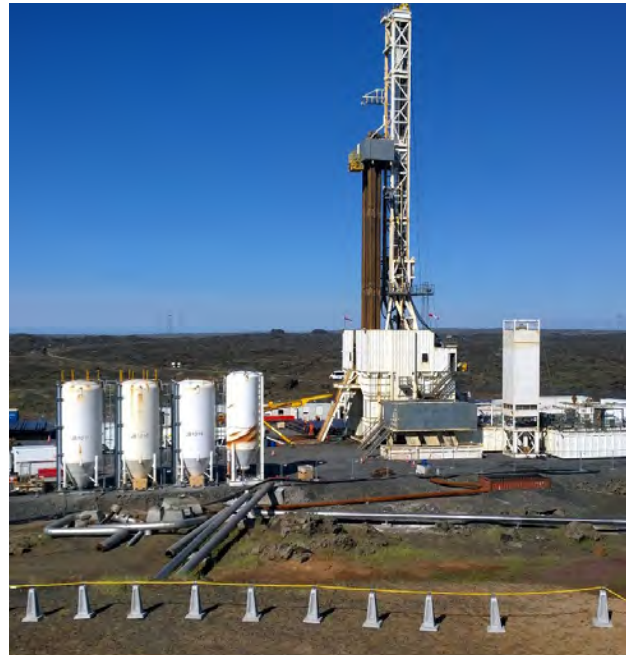
IDDP drill rig (source: https://iddp.is/ )
